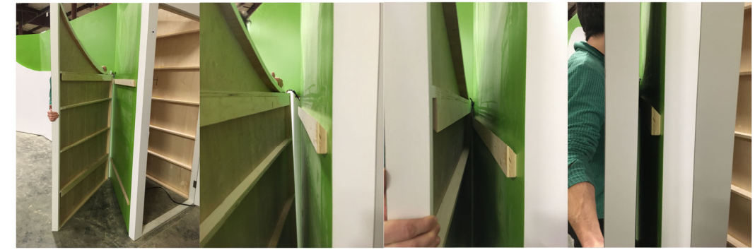
3. LIFT DISPLAY WALL PIECES UP AND ONTO THE WOOD SLATS.
