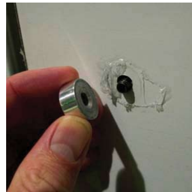
Attach shelf standoff brackets to panel as shown.
